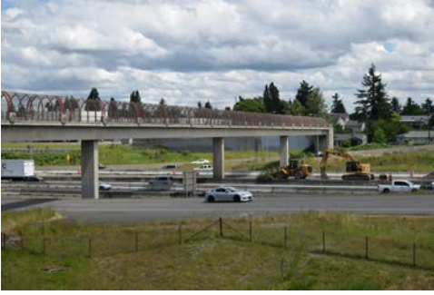
Photo T-11. Bike bridge across I-5.
