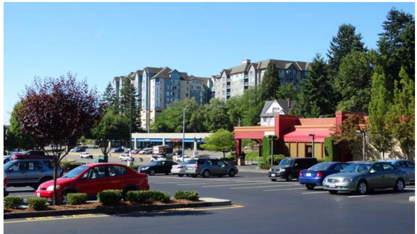
Photo SP-22. Apex Apartments, Mall District.
