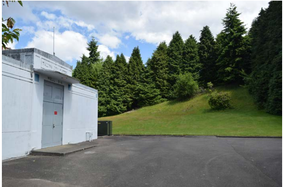
Photo CV-21. Tacoma Public Utilities well site in Northwest District.
