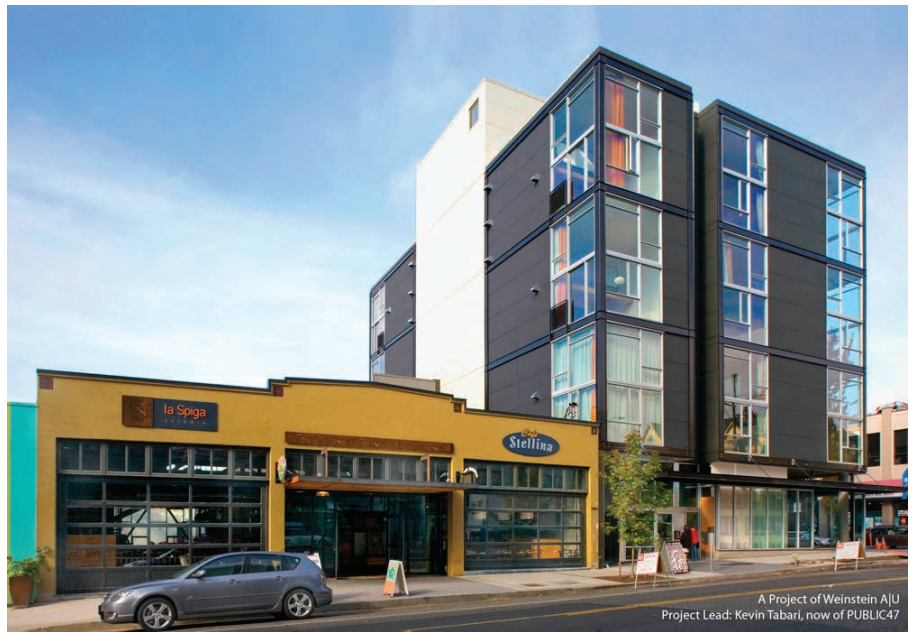
Photo LU-10. Loft infill development.
