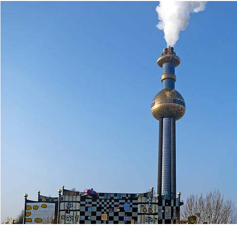
Photo US-5. Fuel and Power Generation Garbage Incinerator reimagined by famous artist Friedensreich Hundertwasser, Vienna Austria.
