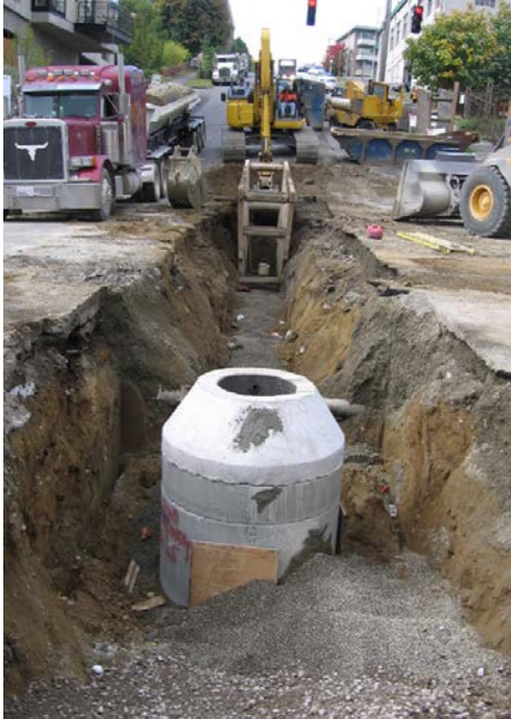
Photo IMPL-1. Street Construction.
