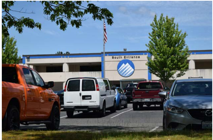
Photo SP-16. Pierce County Annex .
