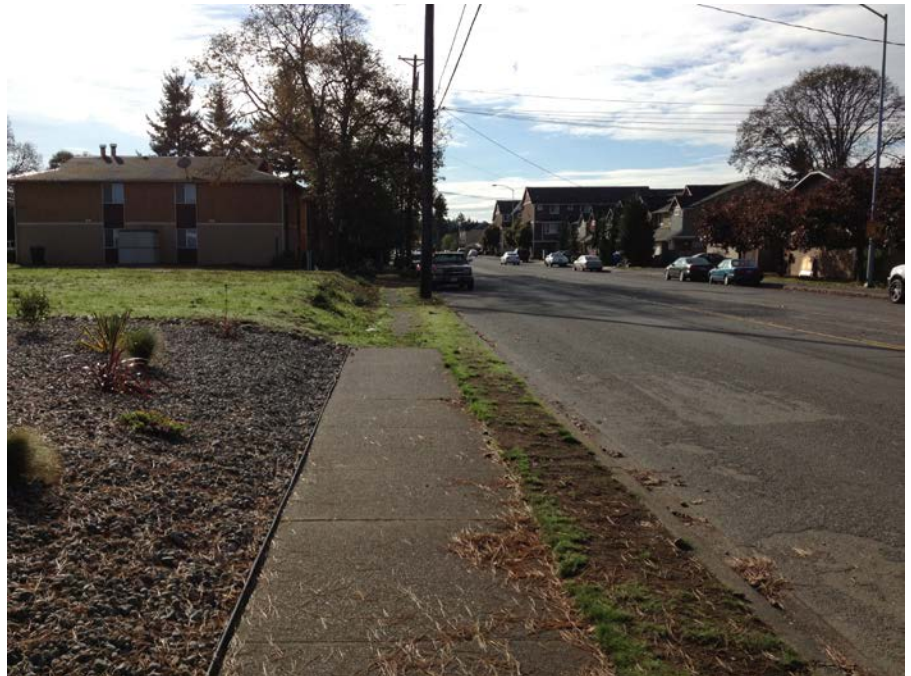
Photo T-5. Incomplete sidewalk in the Madison District.
