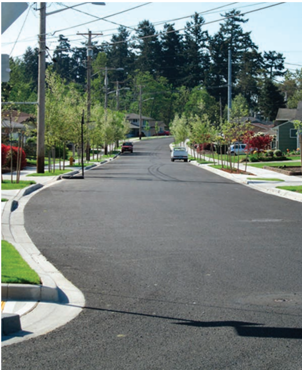
Photo E-4. Permeable pavement roadway (Wapato St, Tacoma).
