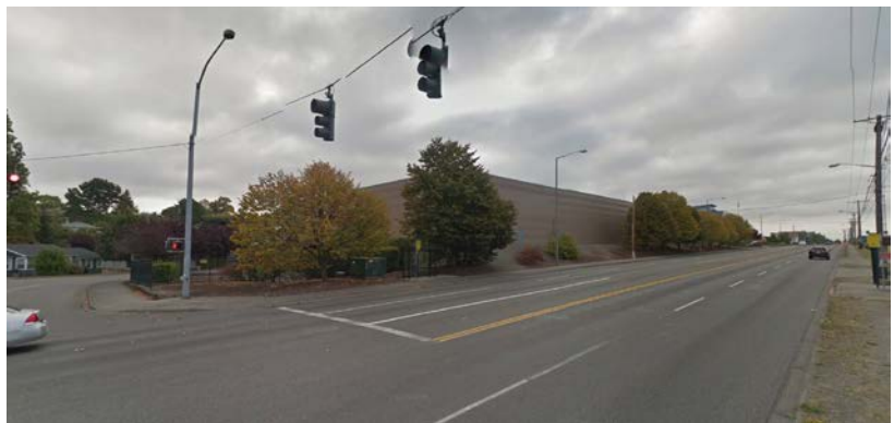
Photo SP-18. City of Tacoma Fleet Services Building, facing S. Pine St.
