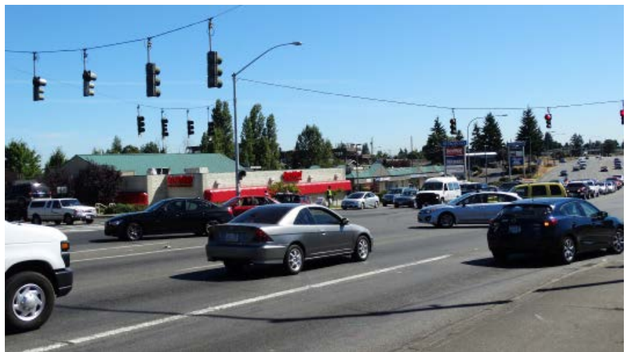
Photo T-9. 38 th Street has a high number of driveways connecting adjacent sites, which impacts negatively on traffic flow and pedestrian safety.
